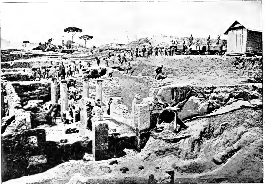
Excavation in Progress
